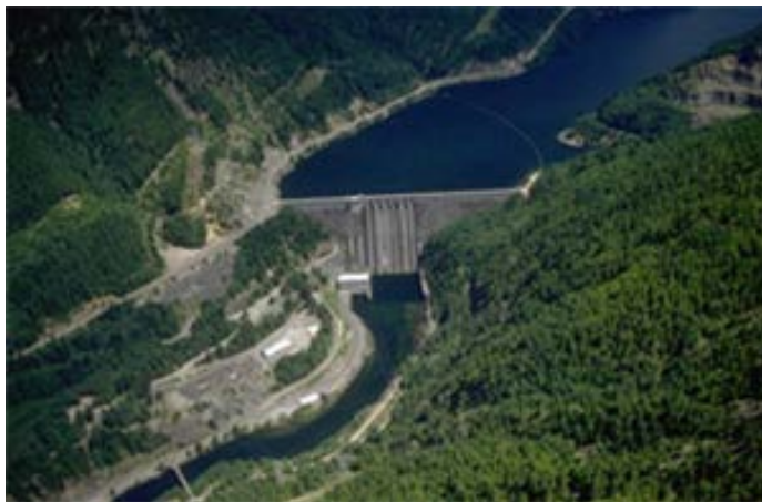
Figure 27. Aerial photo of Detroit Dam, courtesy of the Corps of Engineers.
