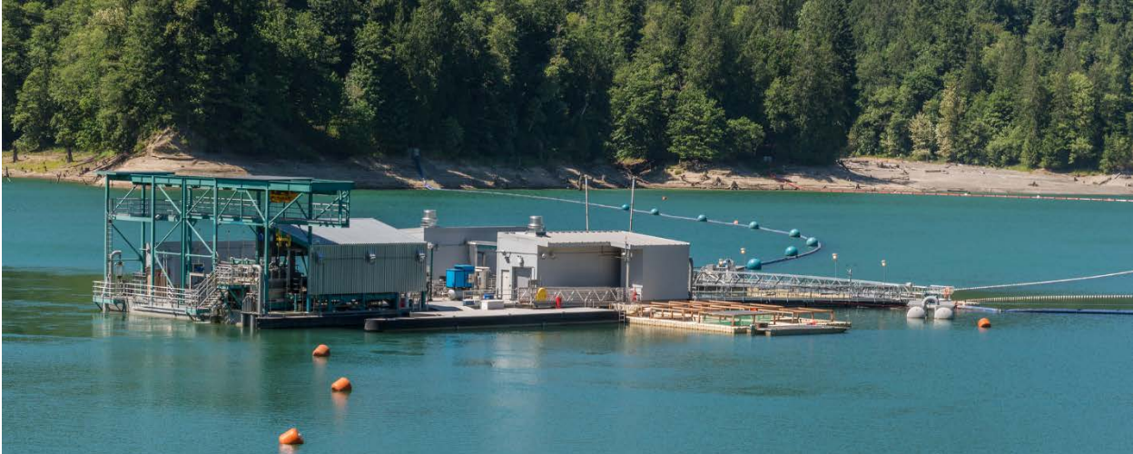
Figure 7. The floating surface collector at Lower Baker Dam. (Photo courtesy of Tony Grover)
