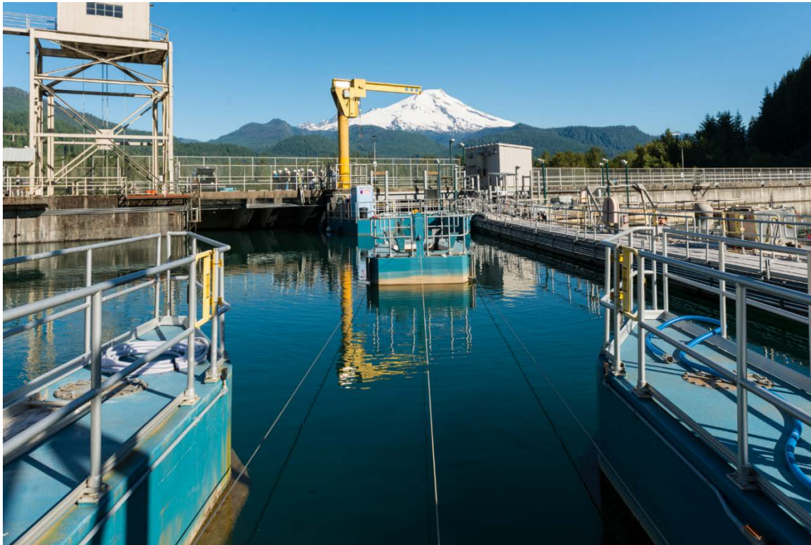
Figure 10. The juvenile salmon transport barge used at Upper Baker to transfer the tank of collected juveniles from the collection facility to a transportation truck via a mechanical pulley system. (Photo courtesy of Tony Grover)
