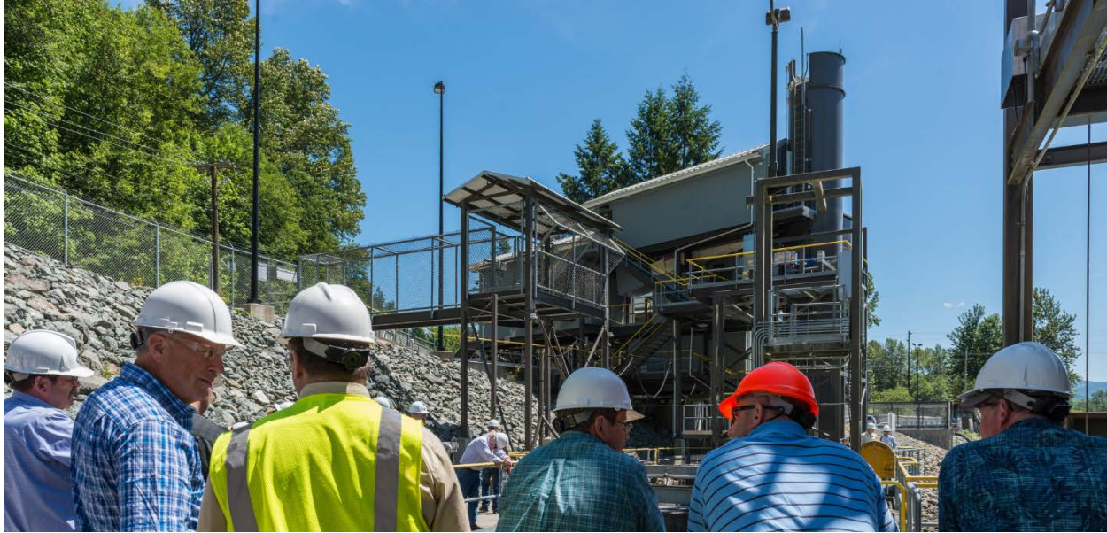
Figure 11. The fish elevator (gray tower on the right) at the adult trap downstream of Lower Baker Dam. (Photo courtesy of Tony Grover)
