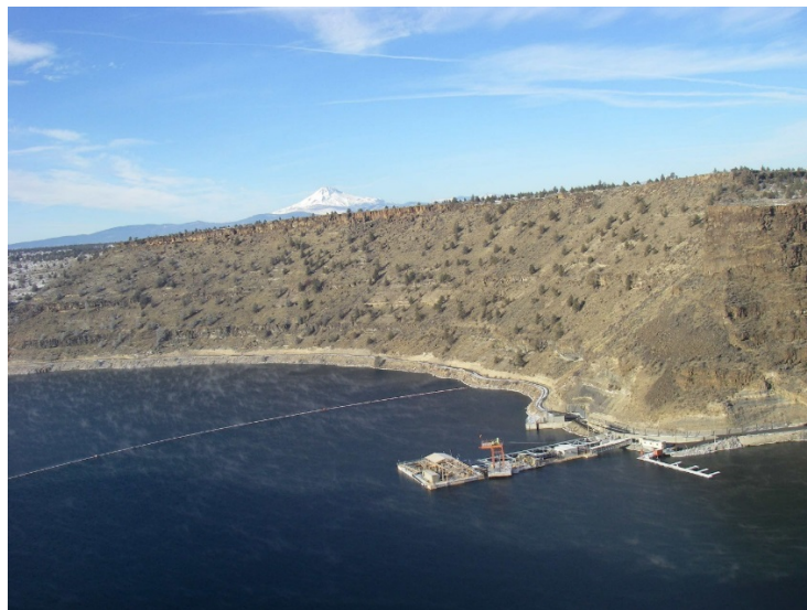
Figure 21. Overview of the Pelton Round Butte surface collector and selective water withdrawal tower. (Photo courtesy of Portland General Electric)
