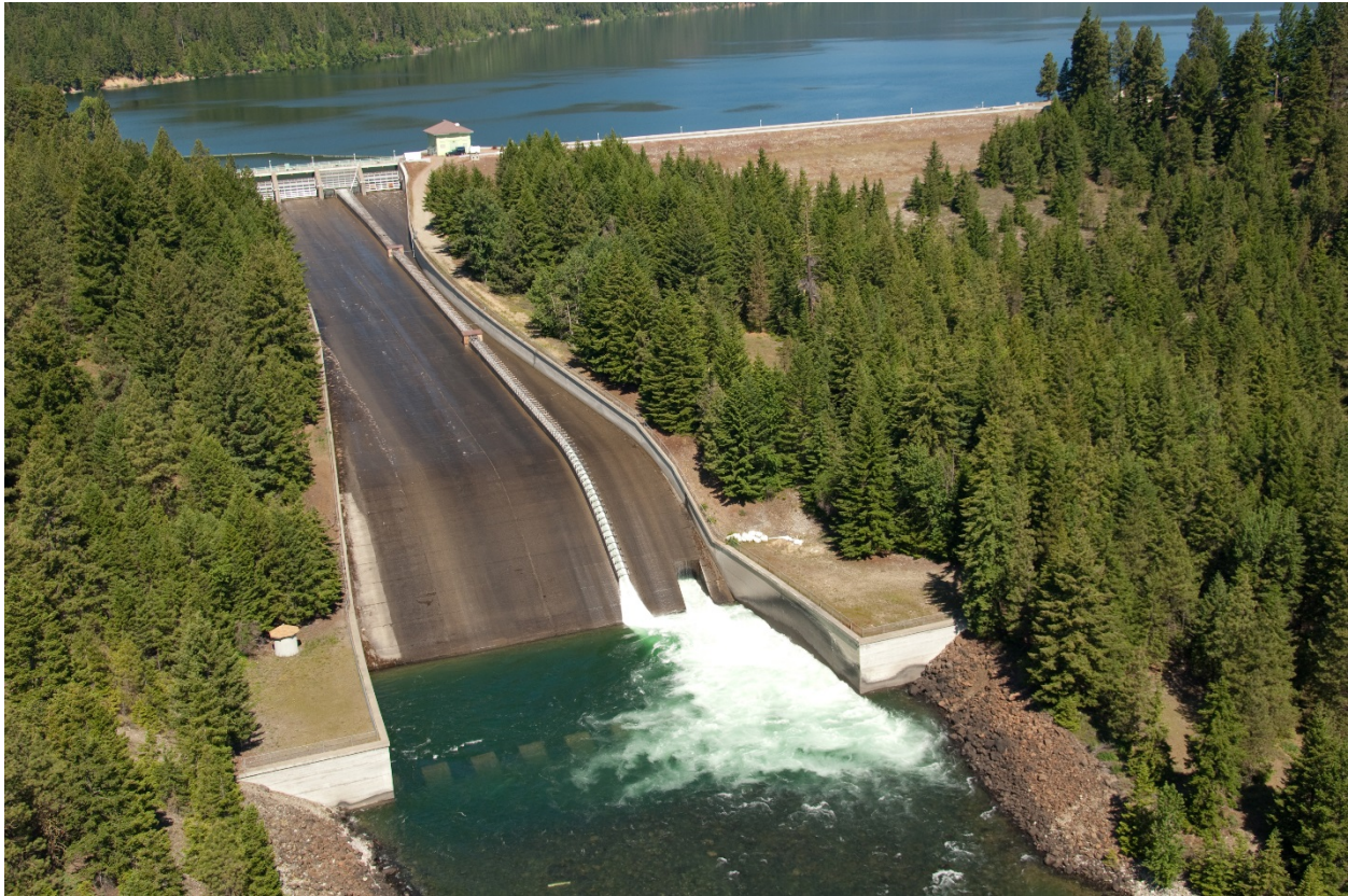
Figure 33. The interim bypass flume on the Cle Elum spillway. (Source: USBR)
