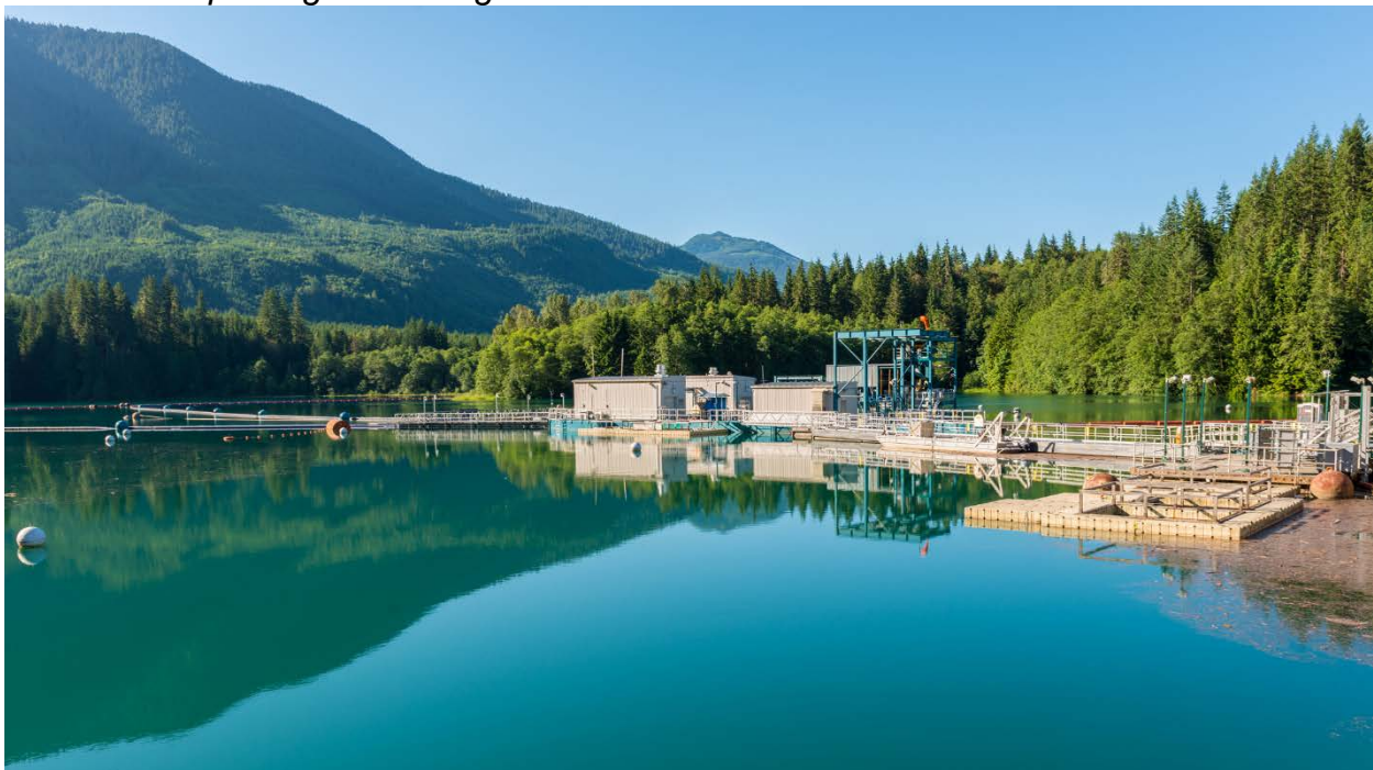
Figure 6. The floating surface collector at Upper Baker Dam. (Photo courtesy of Tony Grover)
