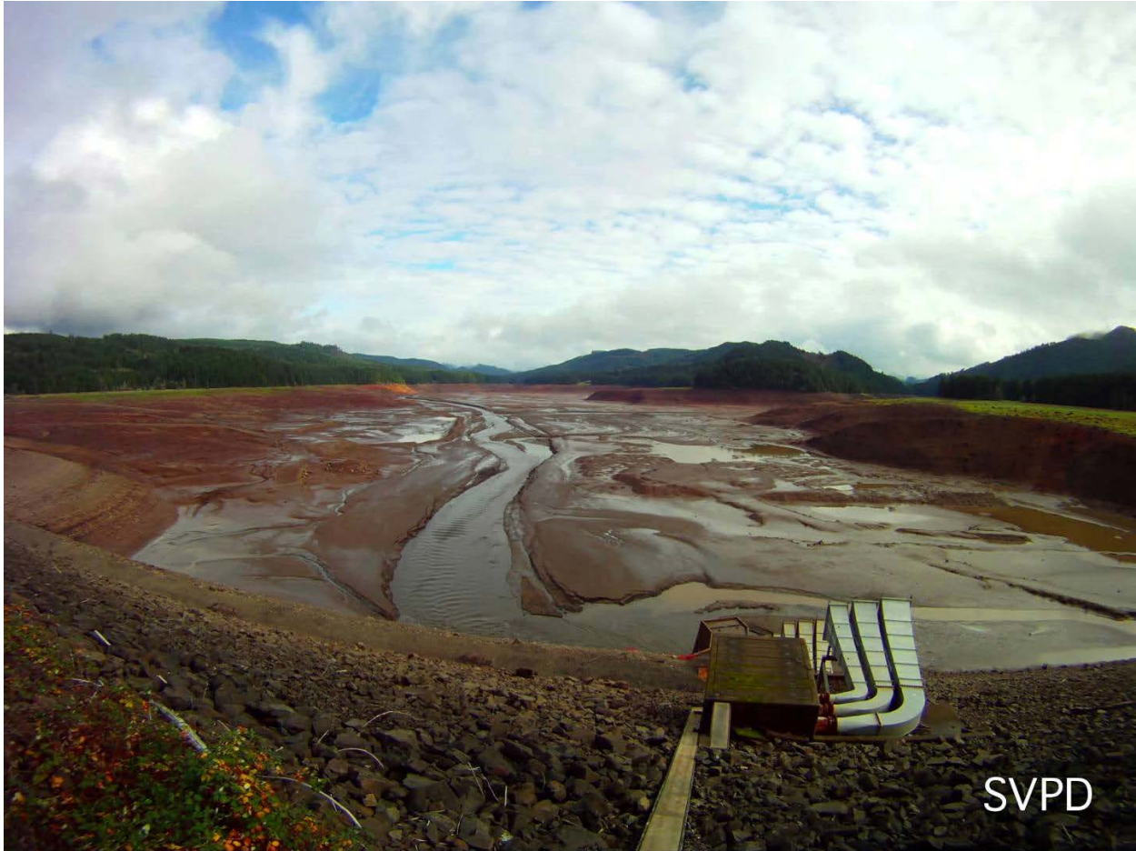
Figure 4. Fall Creek deep drawdown operation (Photo courtesy of Corps of Engineers)
