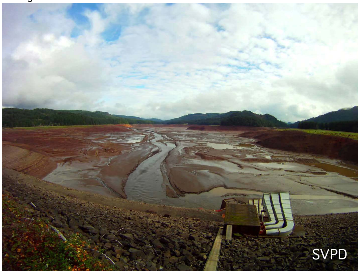
Figure 32. Fall Creek drawdown conditions. (Photo courtesy of the Corps of Engineers)
