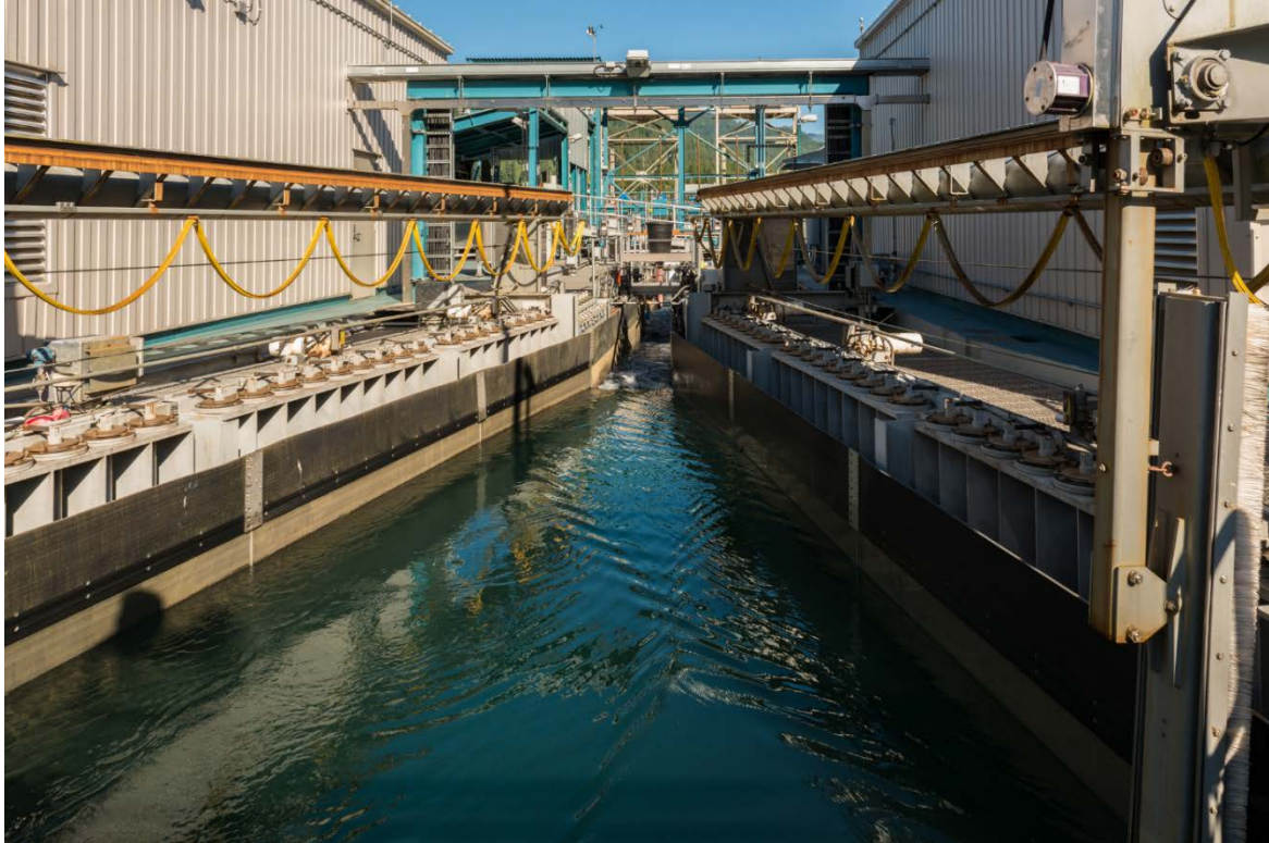
Figure 8. Attraction flow through the concentration flow structure guides the juvenile fish into the collector at Upper Baker. (Photo courtesy of Tony Grover)
