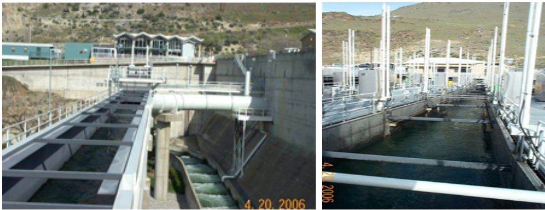
Figure 3. Rocky Reach Dam surface collector and bypass system. Photos courtesy of Chelan County PUD.
