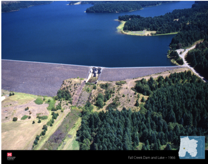
Figure 29. Aerial photo of Fall Creek Dam. (Photo courtesy of the Corps of Engineers)
