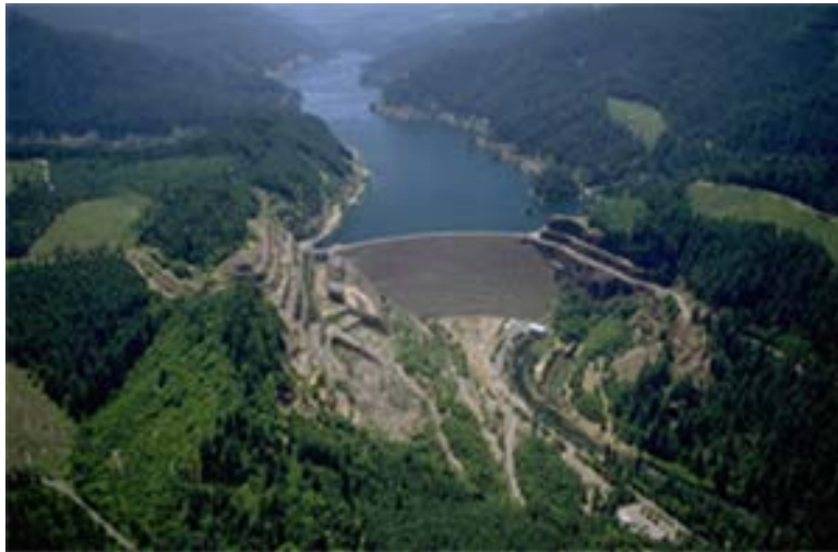
Figure 25. Aerial photo of Cougar Dam. (Photo courtesy of the Corps of Engineers)
