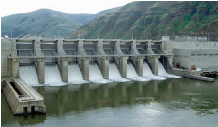
Lower Granite Dam, here spilling water to aid juvenile fish passage, is one of four federal dams on the lower Snake River
