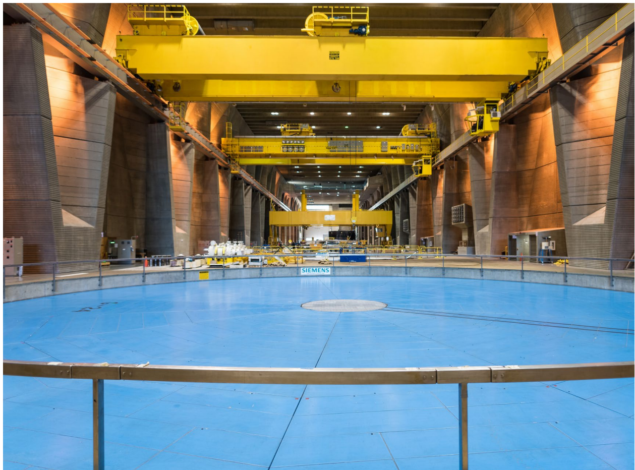
Powerhouse 3 at Grand Coulee Dam, photo courtesy of Tony Grover
