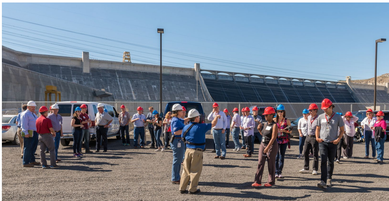
Congressional staff preparing to tour Grand Coulee Dam, August 2016, photo courtesy of Tony Grover
