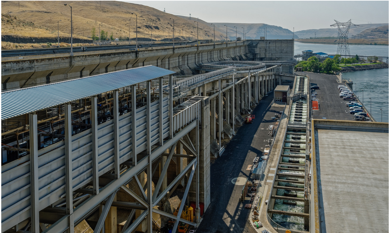
Adult fish ladder and juvenile bypass at Little Goose Dam, photo by Tony Grover
