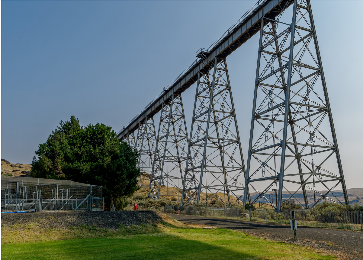
Railroad trestle at Lyons Ferry Hatchery, photo by Tony Grover
