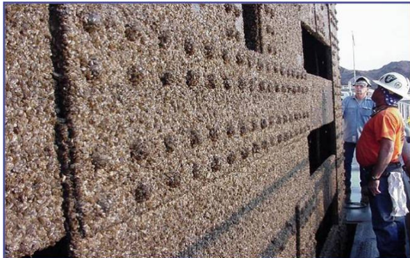
Quagga mussels coating a spillway gate at Davis Dam. Source: USBR.
