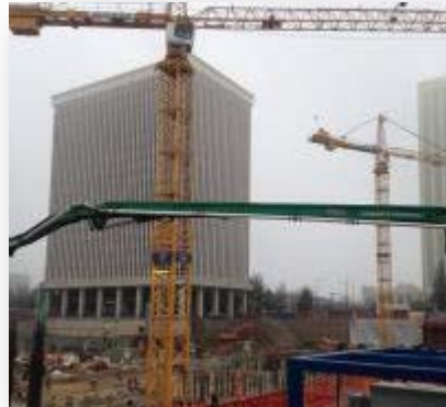
Commercial New Construction
