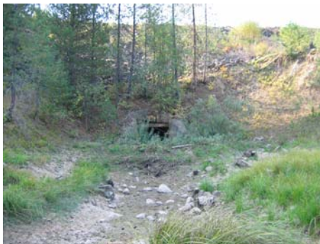
Northern entrance to former Corral Creek box culvert
