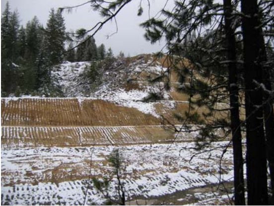
Grading and shaping of hillsides created after removal of Corral Creek box culvert through railroad bed
