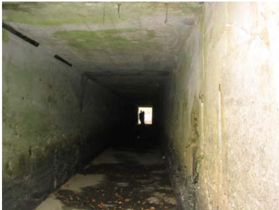
Interior view of former box culvert fish barrier on Corral Creek
