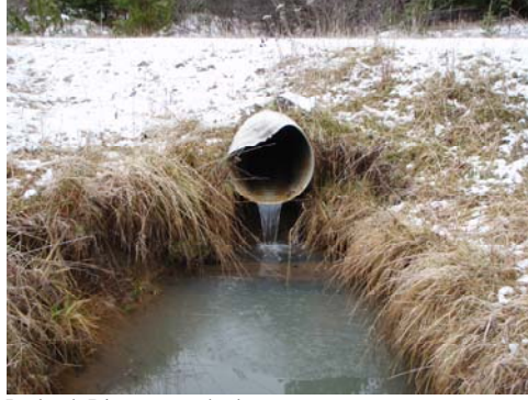
Defective culverts in the East Fork Potlatch River watershed
