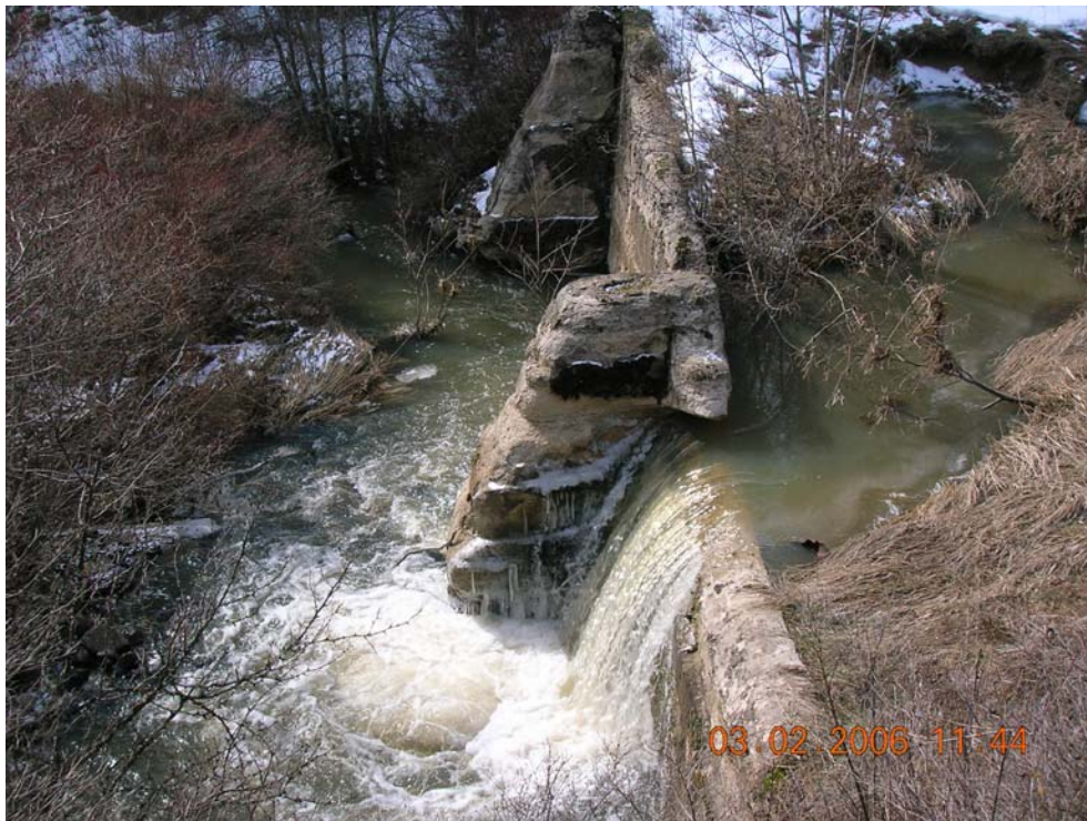
Fish passage barrier created by the remnants of old Troy reservoir dam on West Fork Little Bear Creek
