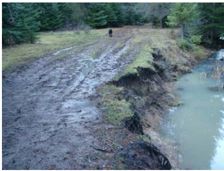
Channelized stream segments along improperly placed road and abandoned railroad bed.
