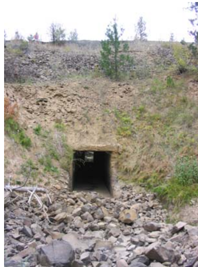
Southern outlet of former Corral Creek culvert
