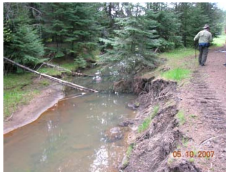
Channelized stream segments along improperly placed road and abandoned railroad bed.
