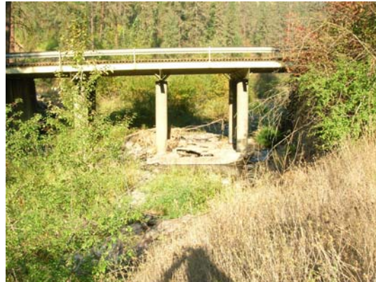
Pine Creek bridge near confluence with Potlatch River
