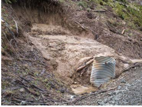
Defective culverts in the East Fork Potlatch River watershed
