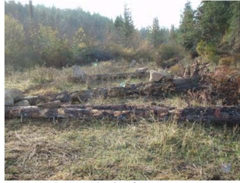
Revegetation in a former scour area
