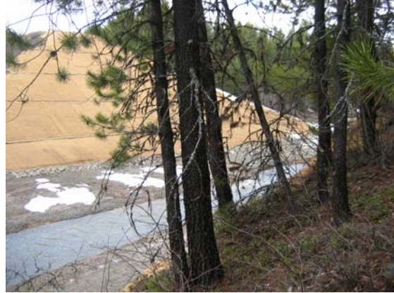
Grading and shaping of hillsides created after removal of Corral Creek box culvert through railroad bed
