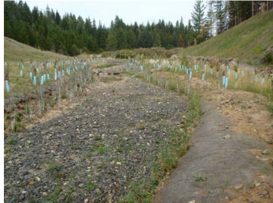
Post construction revegetation of Corral Creek where railroad bed box culvert once existed as a fish migration velocity barrier
