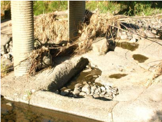
Seasonal out-migration barrier at Pine Creek bridge
