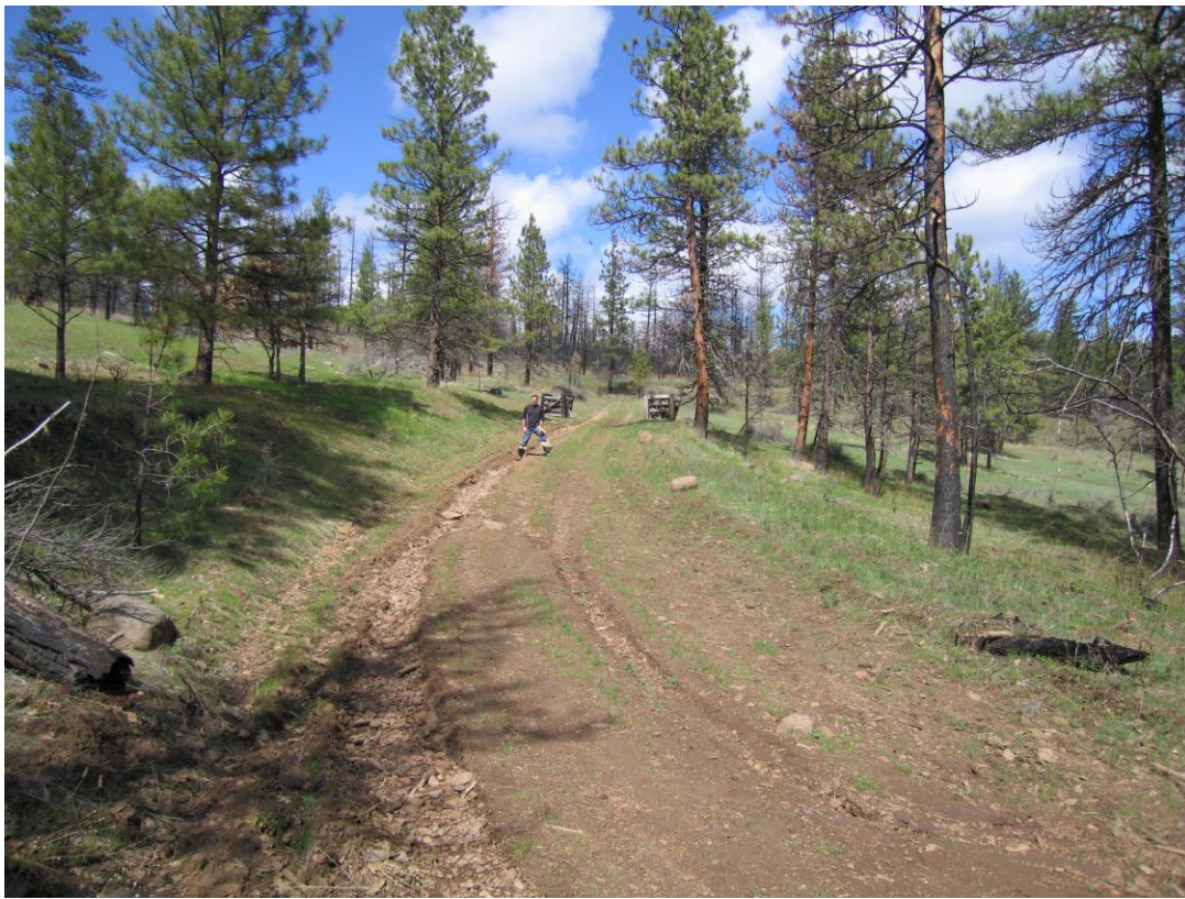
Figure 14. Example of a road showing surface erosion in the Coyote Creek Subwatershed, lower Deschutes River Subbasin, Oregon.
