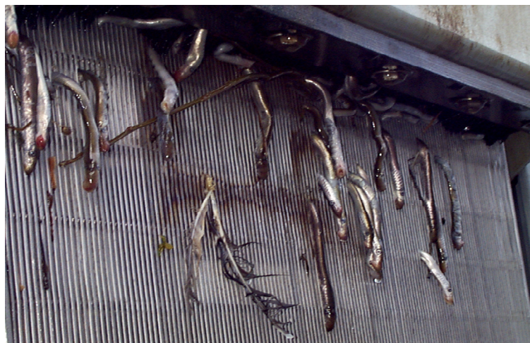
Figure 4. Juvenile lamprey impinged on a mainstem dam turbine screen (CRITFC 2008).
