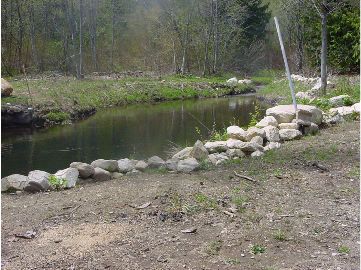
Figure F-1. The Rohlfig coho acclimation pond on Nason Creek is an example of a small pond constructed on a small seasonal stream.
