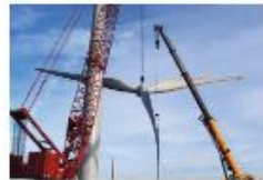
Step 7: Attach the Nacelle & Turbine Blades
