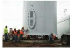
Step 5: Attach Base to Tower Foundation
