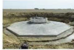
Step 3: Concrete is Poured
