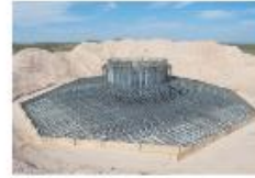
Step 2: Foundation is Started
