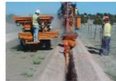
Step 8: Underground Cables are Trenched In
