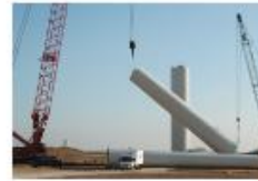
Step 6: Complete Erecting the Tower
