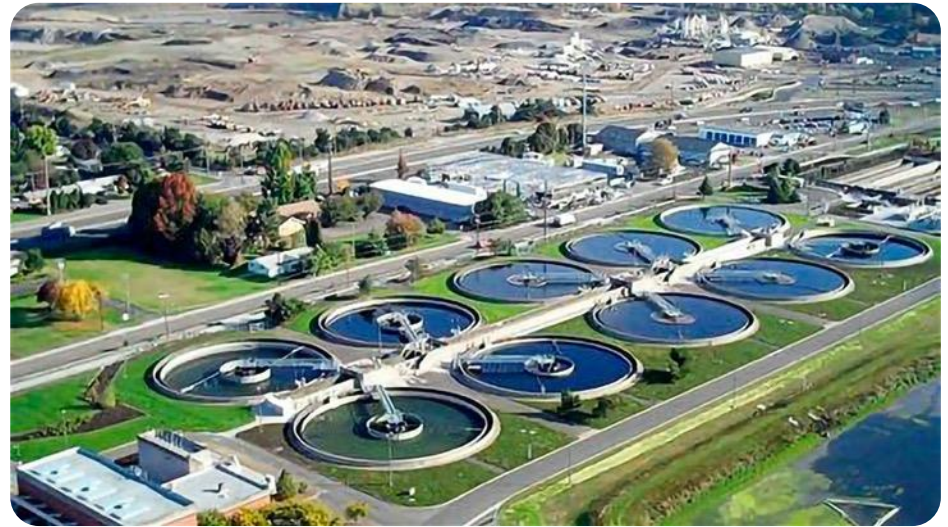
Eugene-Springfield Water Pollution Control Facility
