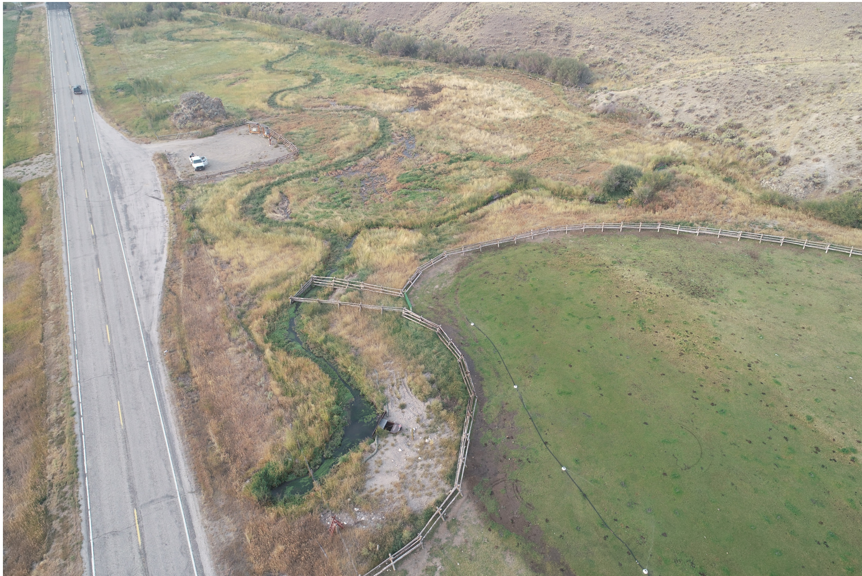
Project area after stream rehabilitation.
