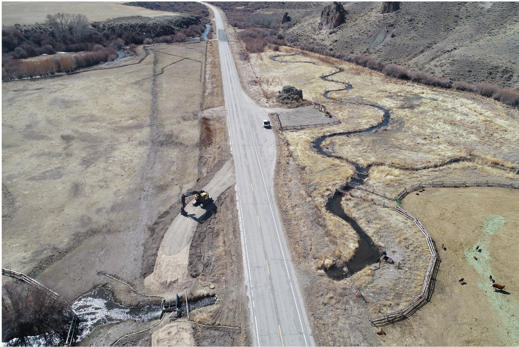
Beginning construction on bypass road for culvert replacement.
