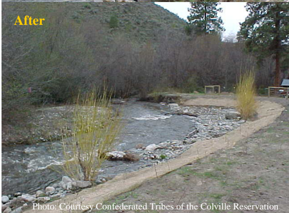
Example of resloping and revegetation techniques implemented in Omak Creek by the Confederated Tribes of the Colville Reservation to reduce streamside erosion.
