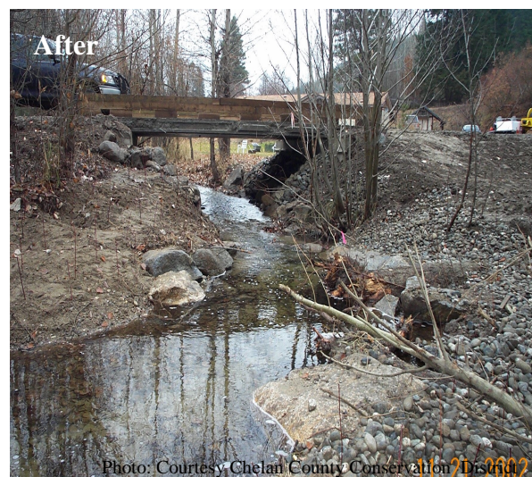
Using bridges (above) and bottomless culverts, the Chelan County Conservation District replaced eight culverts that were barriers to anadromous fish.
