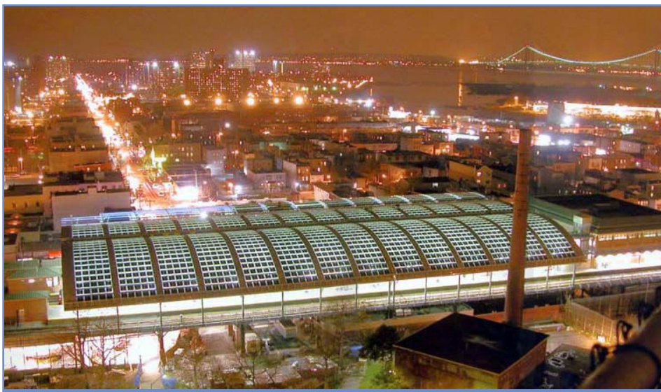
Coney Island’s Stillwell Avenue Terminal is a 76,000 square foot glass and steel structure using an innovative, panelized construction system of semi-transparent photovoltaic modules. These solar modules function both as enclosure and a source of approximately 250,000 kilowatt hours per year in renewable energy, the equivalent of the usage of approximately 40 single family houses.
