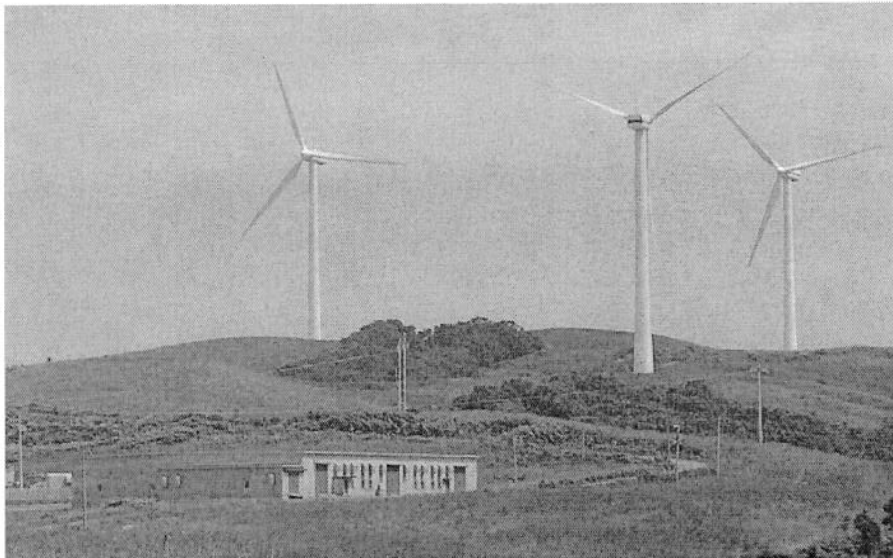
Figure 8. 32MW wind farm using a 4MW 1.5hour with 6MW peak VRB installed in Sapporo Japan to smooth voltage fluctuations caused by wind variations.
