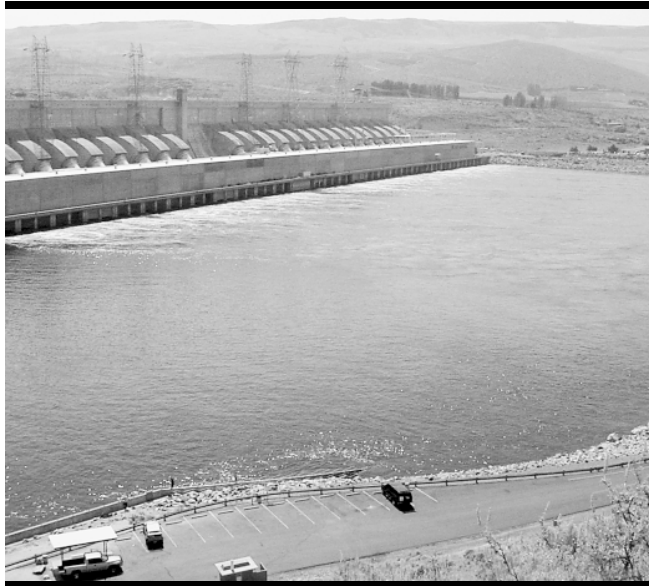
FIGURE 40: Photo Looking Down at Current Parking Facility at Chief Joseph Dam
