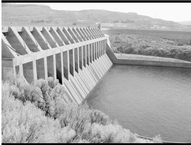
FIGURE 28: Photo Chief Joseph Dam from Right Abutment
