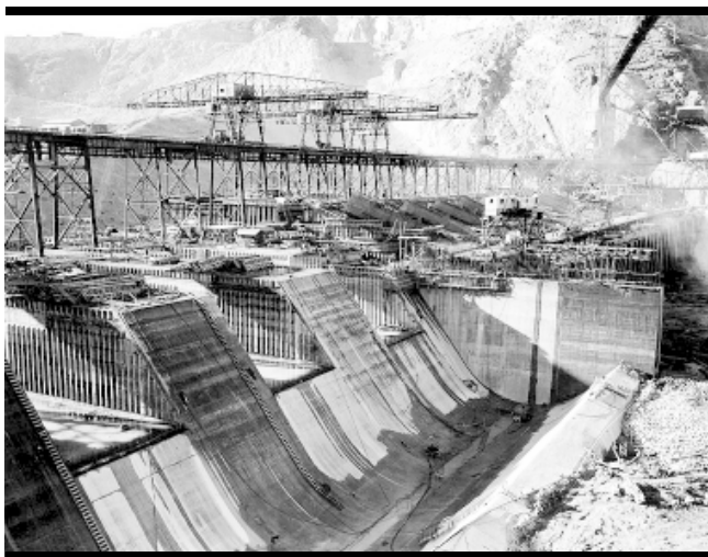
FIGURE 9: Photo of Spillway Construction at Grand Coulee Dam, 1937
