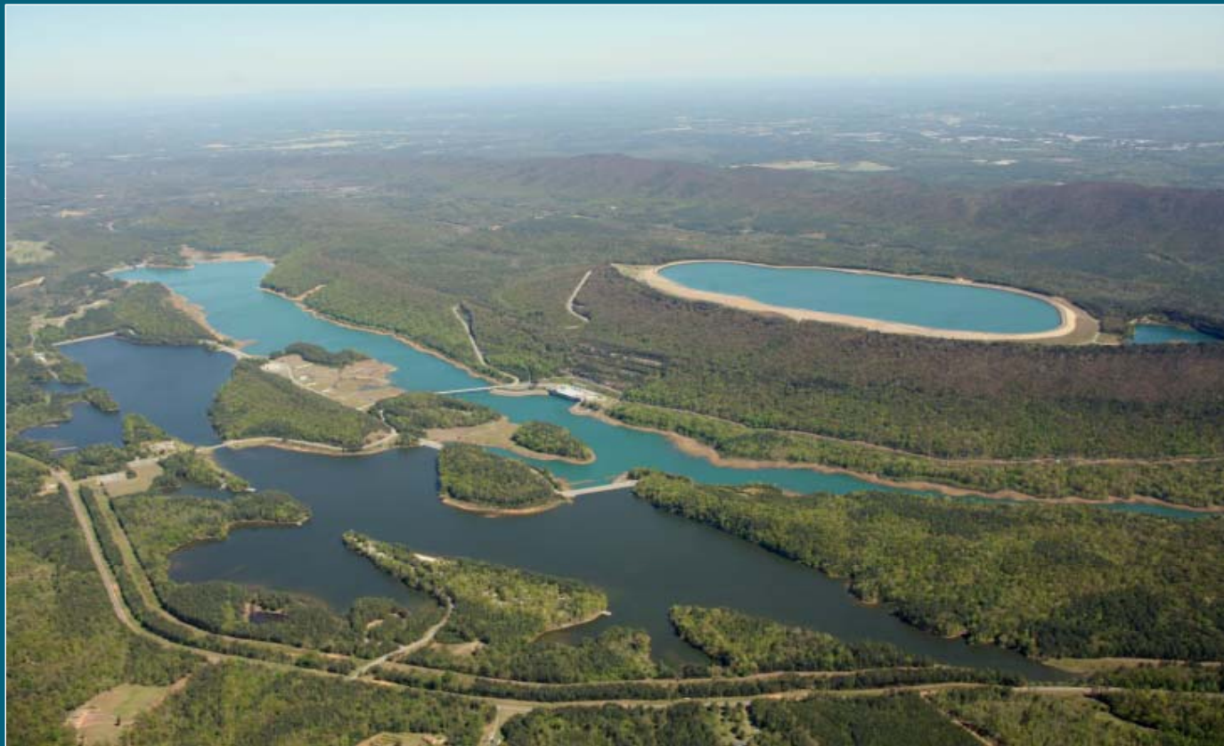
1095-MW Rocky Mountain Pumped Storage Project
