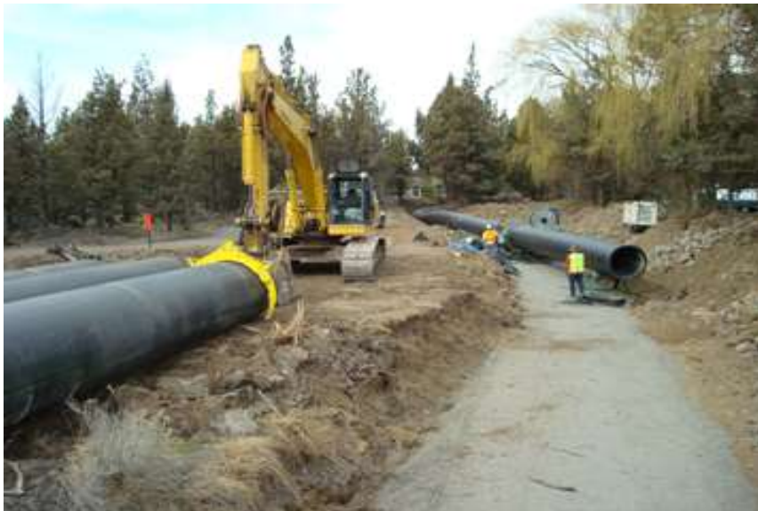
Figure 1: conduit project under construction
