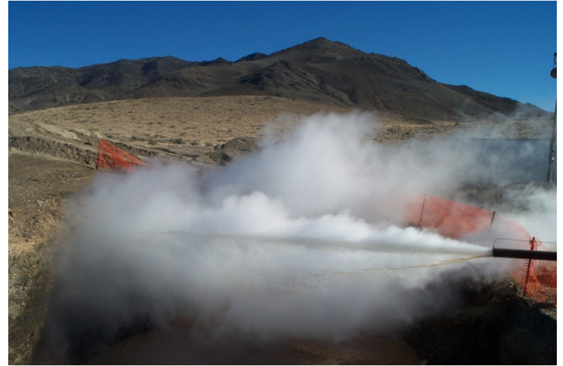
Geothermal well test in the Basin and Range of Nevada
