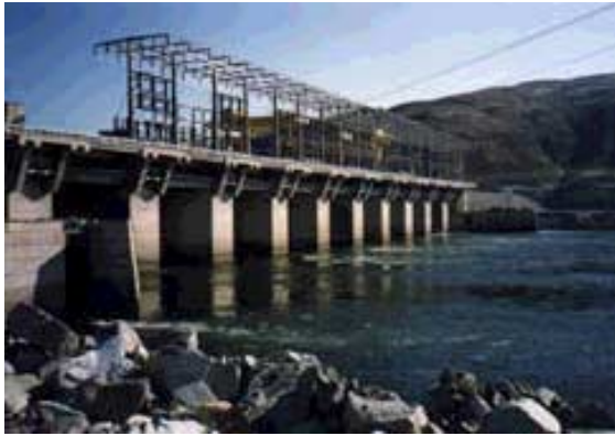
Figure 7.3. Wells Dam, which uses a unique hydrocombine configuration that is thought to contribute to its success in passing juvenile salmonids with low associated mortality. Photo from the US Army Corps of Engineers' Digital Virtual Library.
